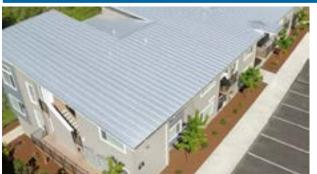
The Clip-Lock<sup>™</sup> Standing Seam delivers a panel with strong clean continuous grace, together with unequaled quality. This provides you a weather tight roof to last a lifetime. Clip system allows for extremely long panels, without the need for laps.
